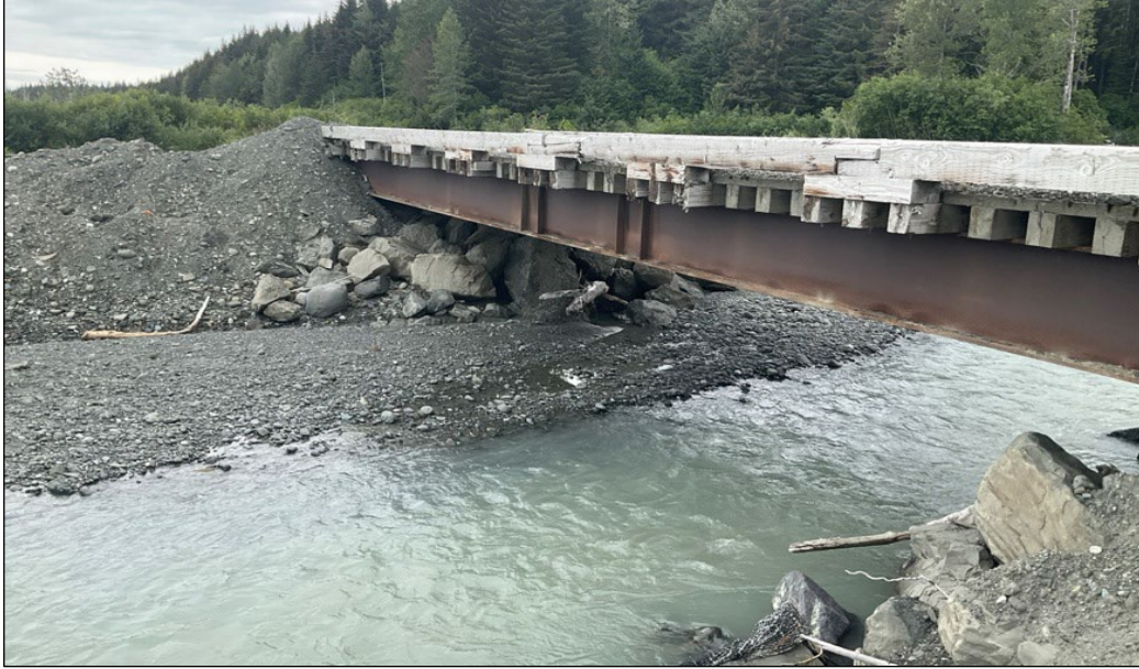
Figure 2.—West abutment of Carson Creek bridge.
