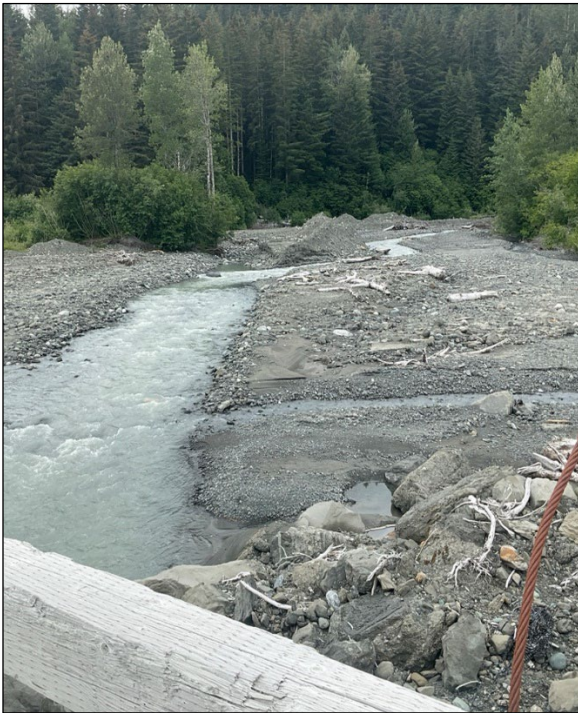
Figure 3.—Berm piles upstream of Carson Creek bridge.
