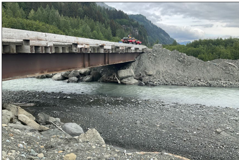
Figure 1.–East abutment of Carson Creek bridge.
